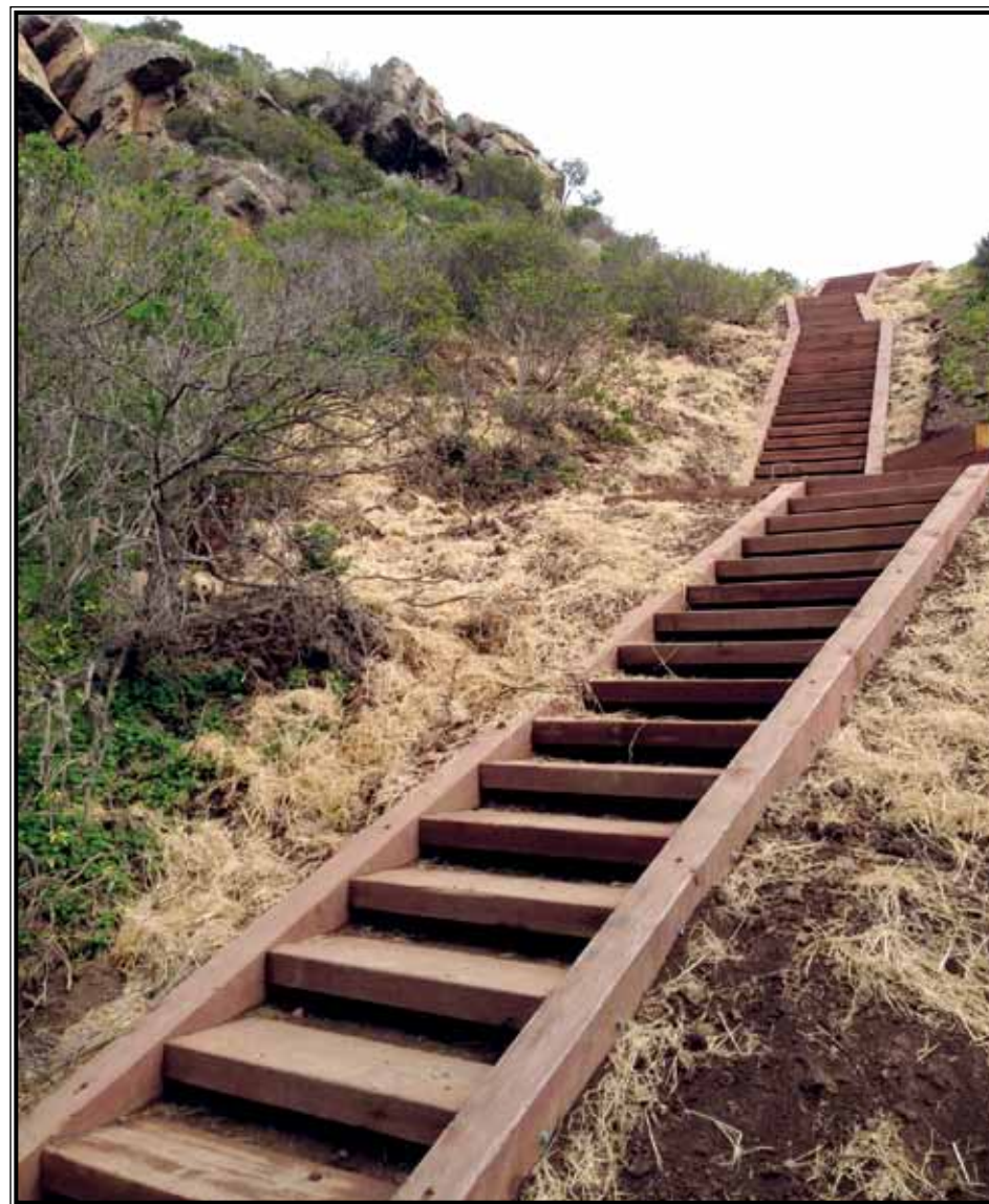
Workers installed stringer steps (above) and box steps (below) on the Saddle Trail.
