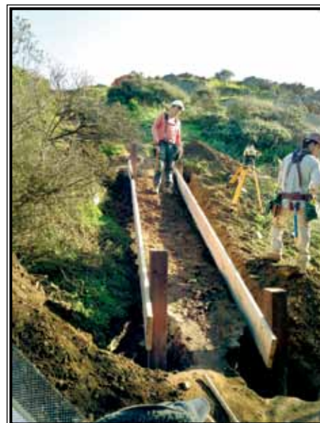
Workers installed stringer steps (above) and box steps (below) on the Saddle Trail.
