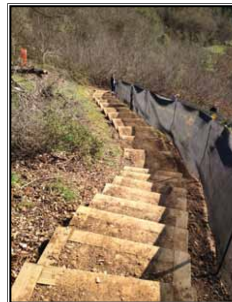
Workers installed stringer steps (above) and box steps (below) on the Saddle Trail.
