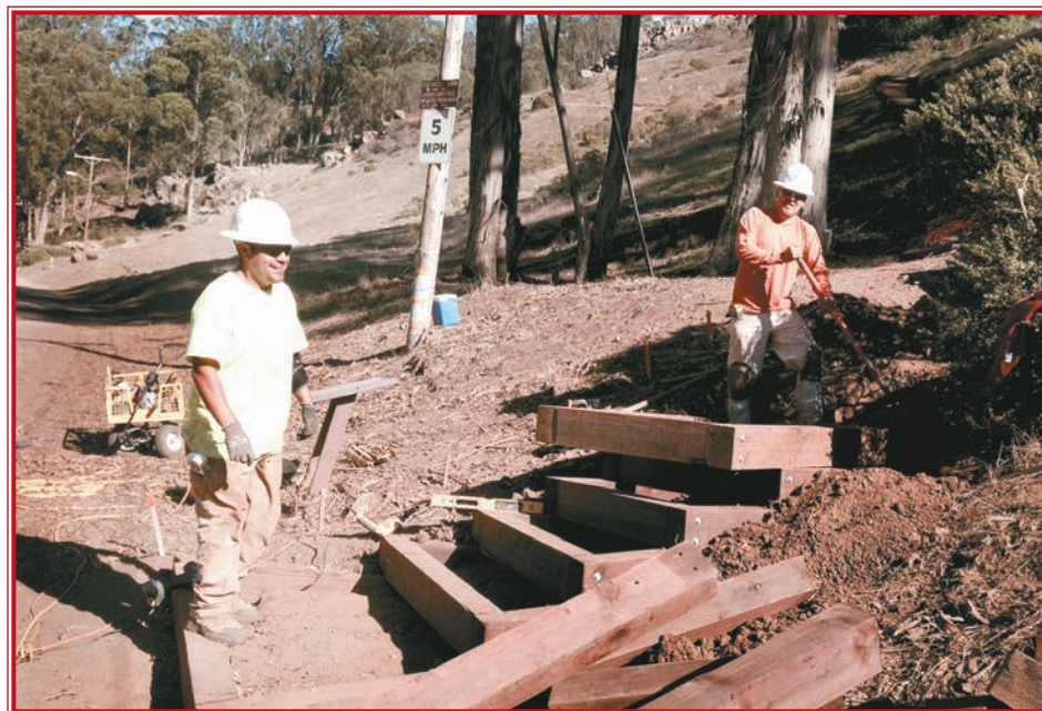
Crews build new railway steps in Glen Canyon.
