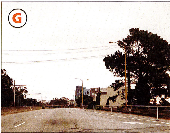
Ramp Entrance onto Northbound San Jose Avenue.
