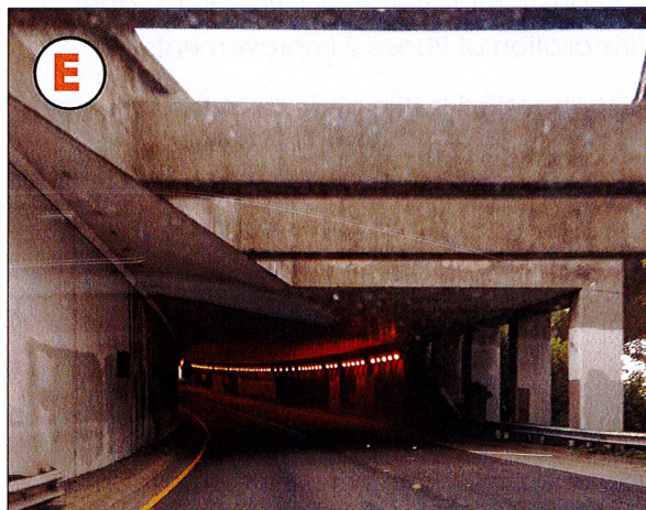
San Jose Avenue Off-ramp Tunnel Under I-280.
