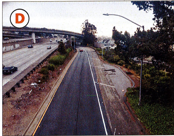
San Jose Avenue Off-ramp Two-to-One Lane Merge.
