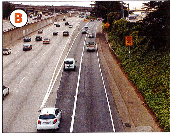
Northbound I-280 north of Baden Street.
