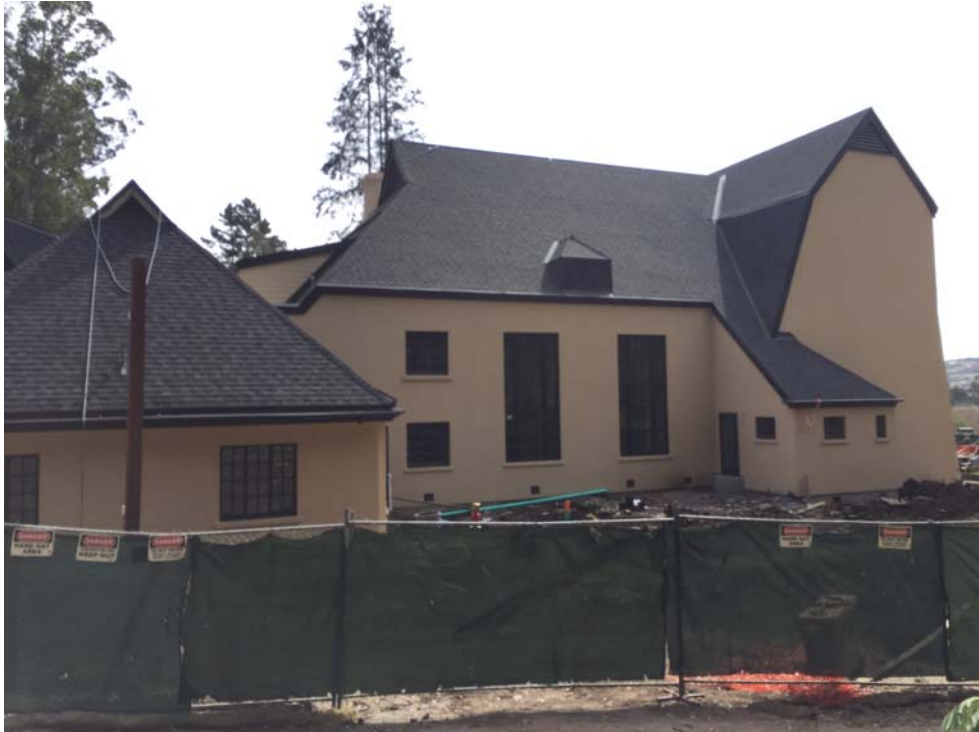
West façade with New Windows, Stucco, and Roof
