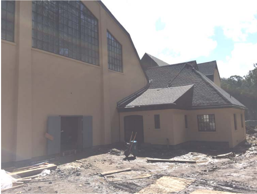
Gymnasium Exterior with New Windows, Stucco, and Roof
