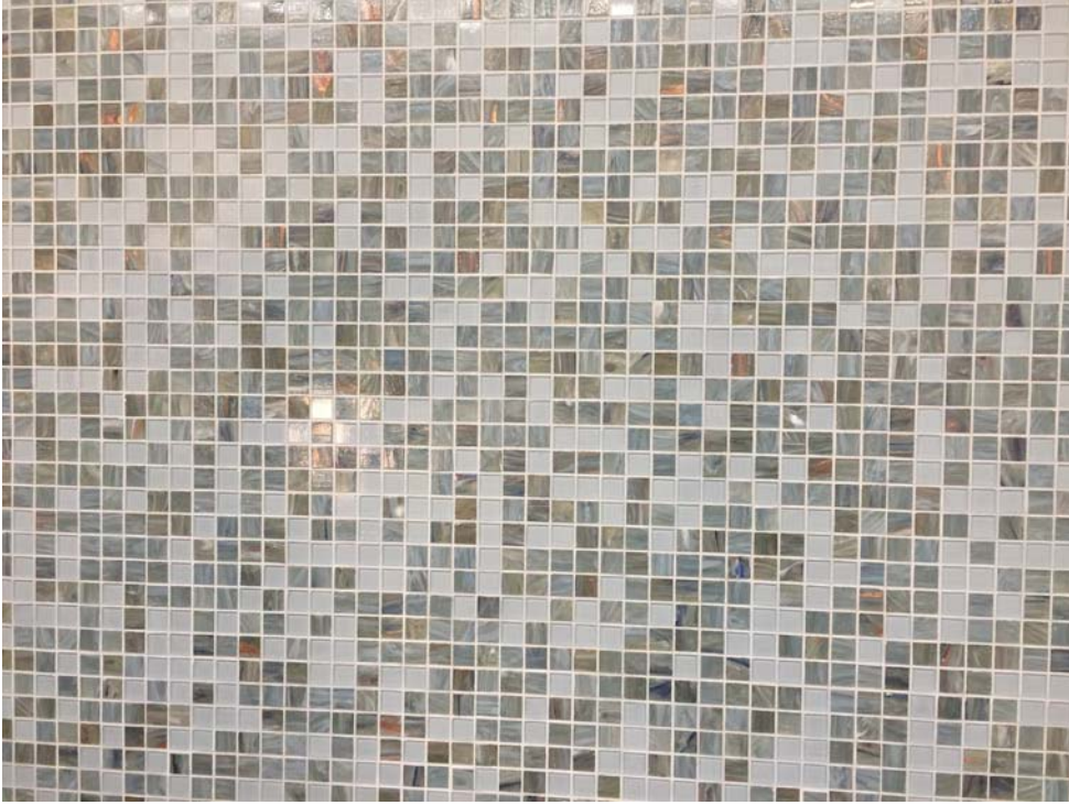
Main Lobby – Mosaic Tile Backsplash at Drinking Fountain
