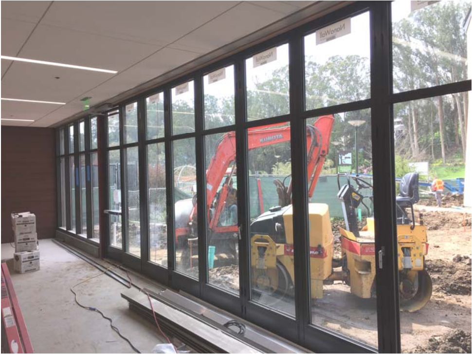
Multi-purpose Room – Folding Glass Wall
