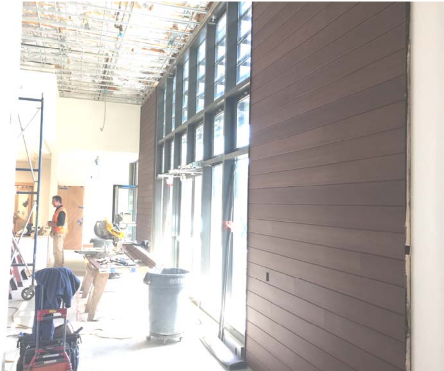
Main Lobby – Entry Doors
