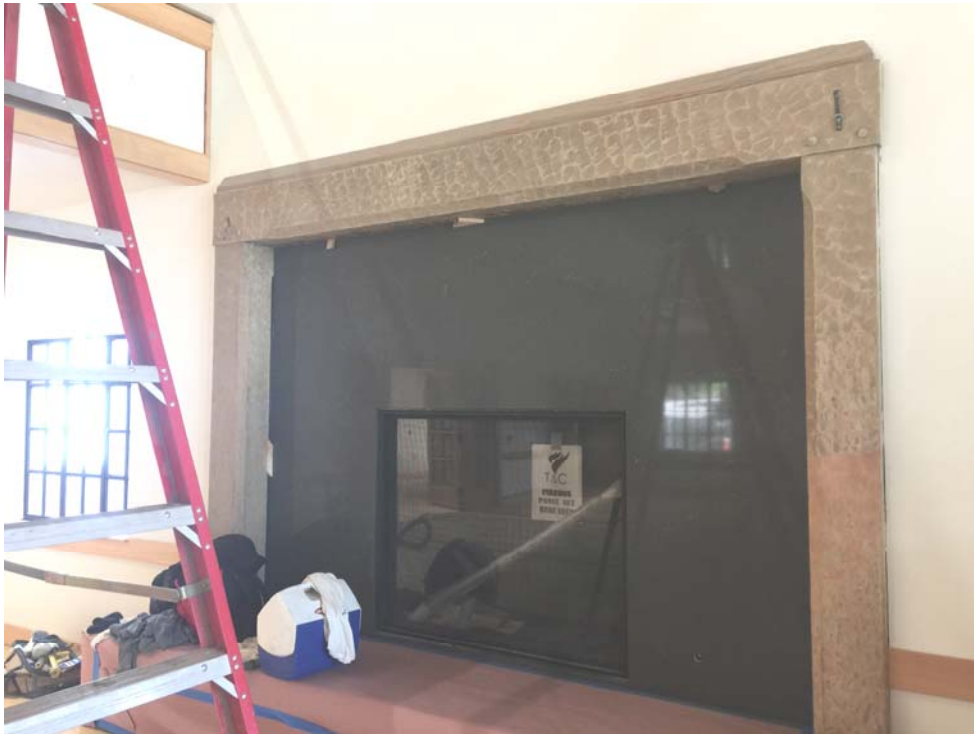
Auditorium Restored Fireplace
