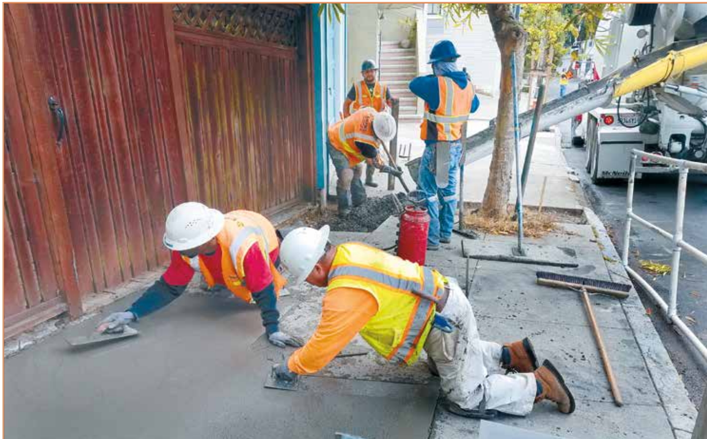
Contractor crews smooth new sidewalk flags on Diamond Street in Glen Park.
