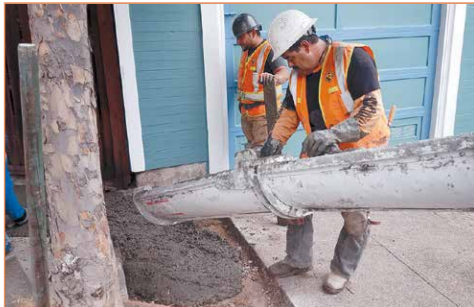
Concrete is poured for new sidewalk squares on Diamond Street.
