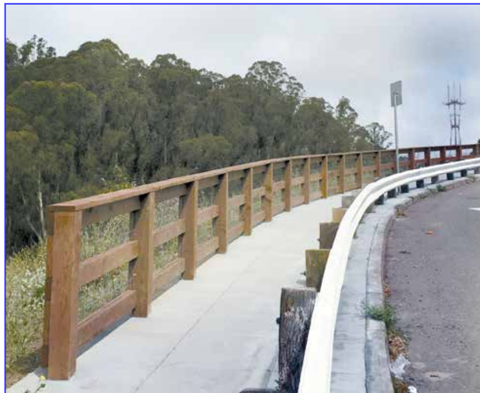
The new guardrail on Diamond Heights Boulevard.
