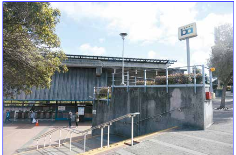
Glen Park BART Station Diamond Street entrance.
