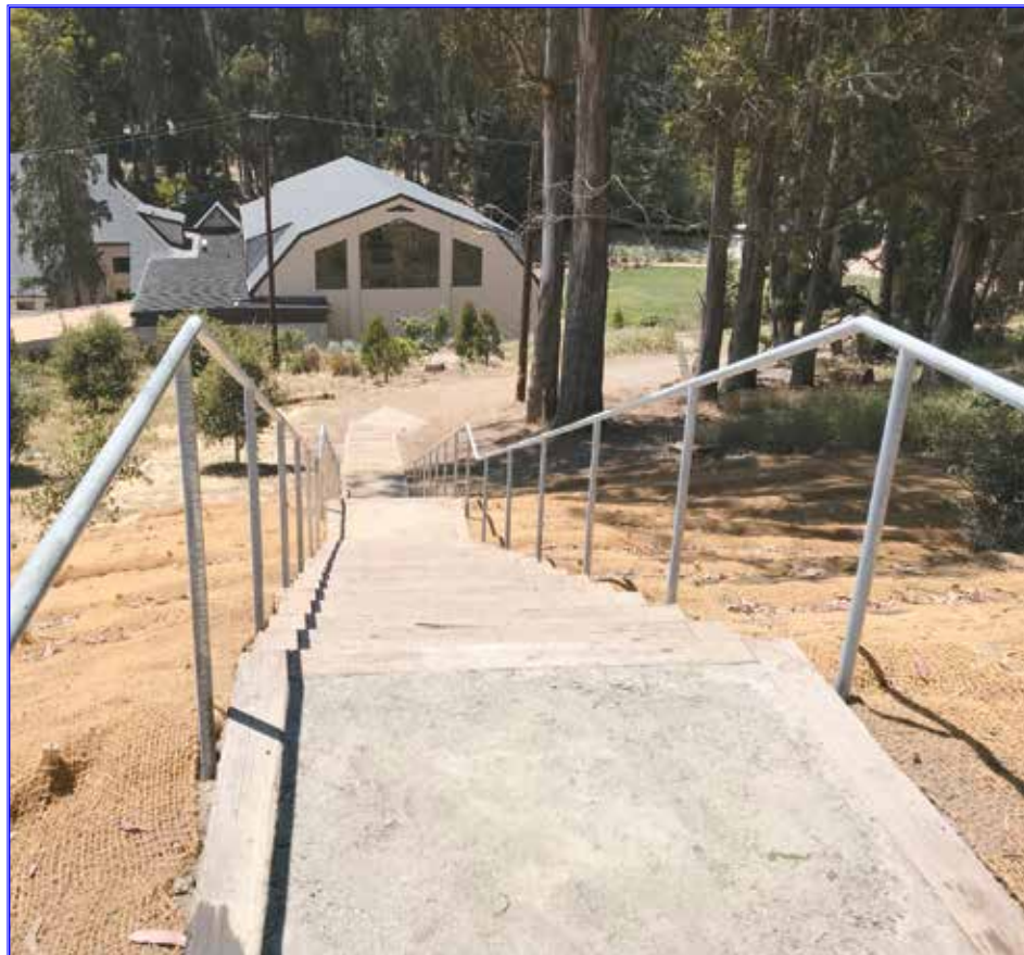
The Sussex Street steps leading into Glen Canyon from Elk Street were completed in June. Photo courtesy of Jeff Sheehy
