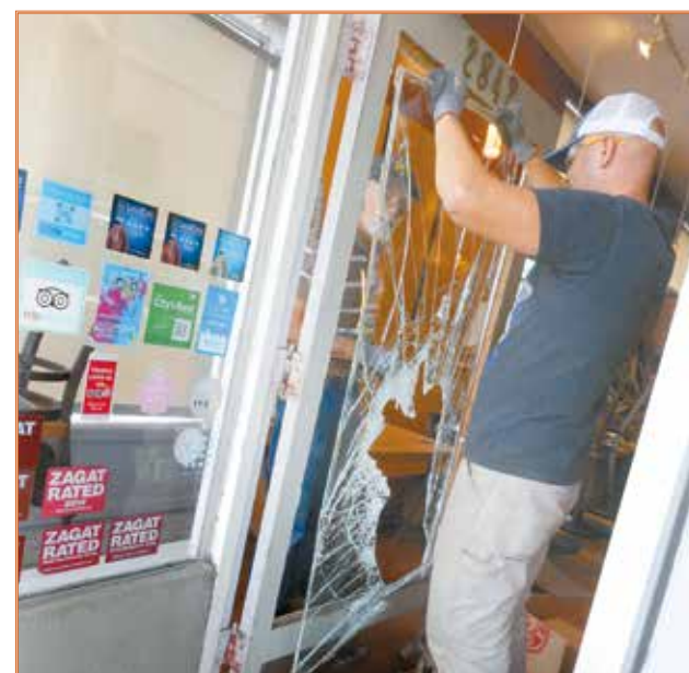
A workman removes the broken door glass at Gialina.
