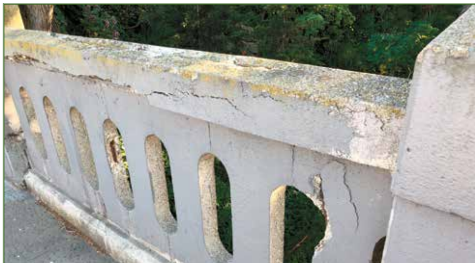
The Richland Bridge over San Jose Avenue, top and its broken railing, above. Photos by Gail Bensinger
